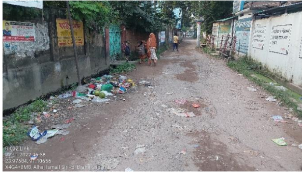
Road-002, Brahmanbaria Paurashava
